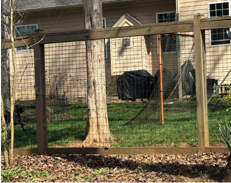
Style 7 -- Wood and Woven wire. Only to be used where not visible from the street
